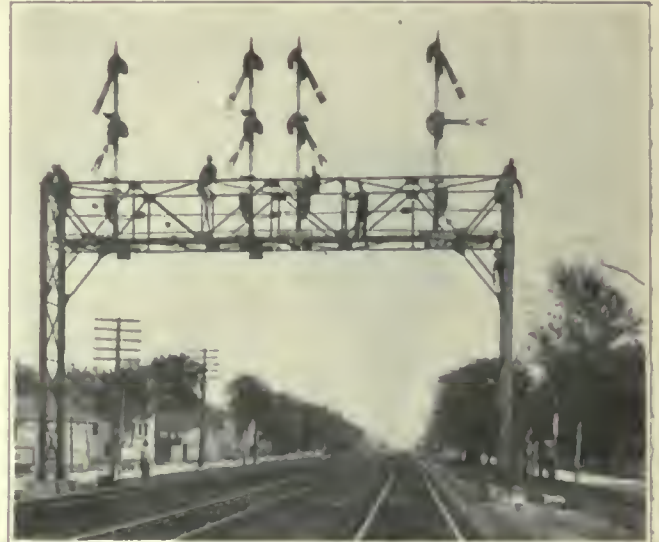
FIG. 288. SIGNALS. Three track signal bridge on the Chicago, Burlington & Quincy Railroad at La Grange, Ill.
